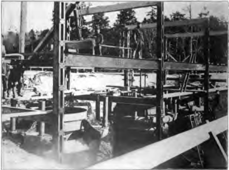
VICTORIA HYDRAULIC COMPRESSOR. Upper End, Showing Air Entraining Tubes.
